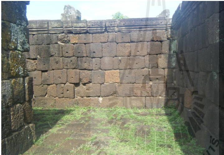
The laterite and sandstones used in the construction of the temple.
