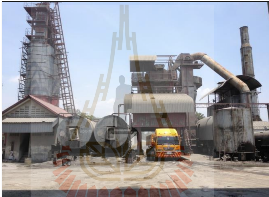
Figure 2.4 The mixing plant of fiber reinforced asphalt concrete
